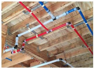
The advantages of PEX tubing for potable hot and cold water systems are detailed in PPI's new TN-31 document.
